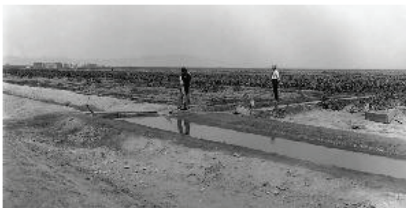
A sewer farm near Salt Lake City, Utah. SOURCE: Utah Historical Society, circa 1908.
