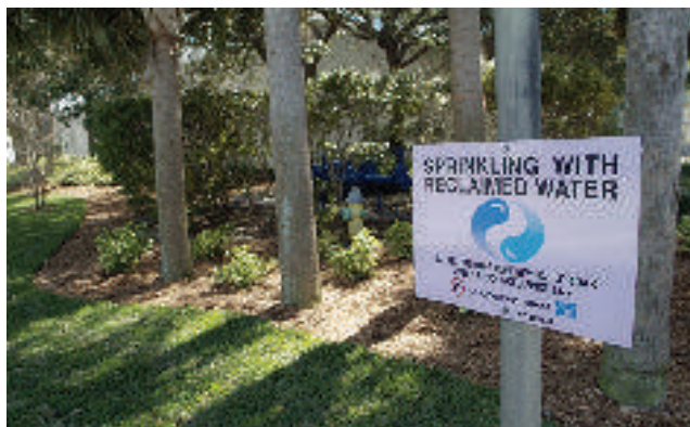
Landscape irrigation with reclaimed water in St. Petersburg.
